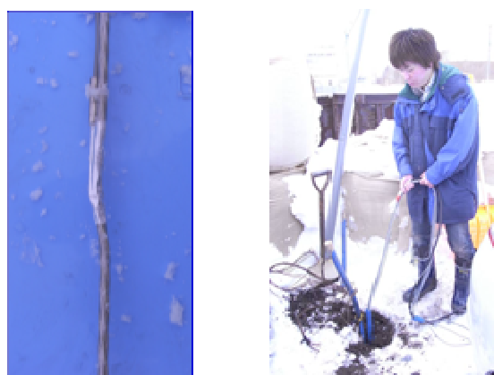
Figure 3.1: Example of hot wire cable (left) and example of installation (right)
