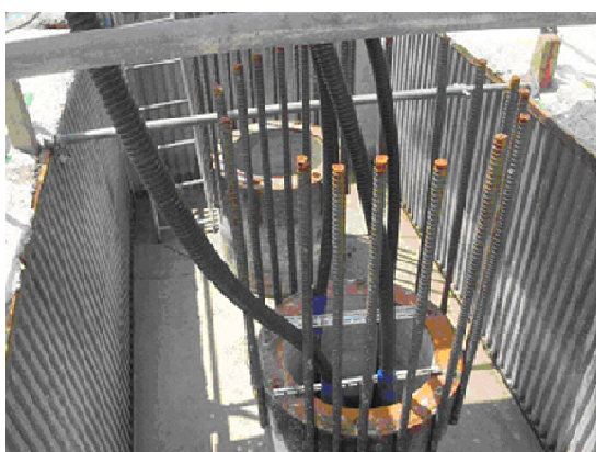
Figure 7.2: Energy pile using pre-casting concrete pile.
