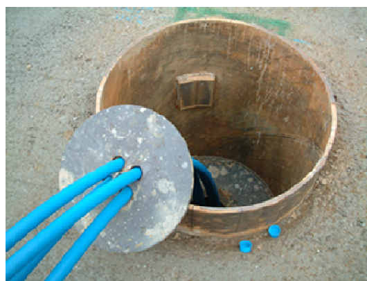
Figure 7.3: Energy pile using steel pile.
