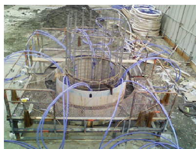
(a) U-tubes inside reinforced frame (b) U-tubes outside reinforced frame
