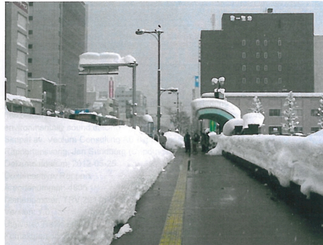
Non-skid winter roads Solar heat and heat storage for environmentally sound deicing
