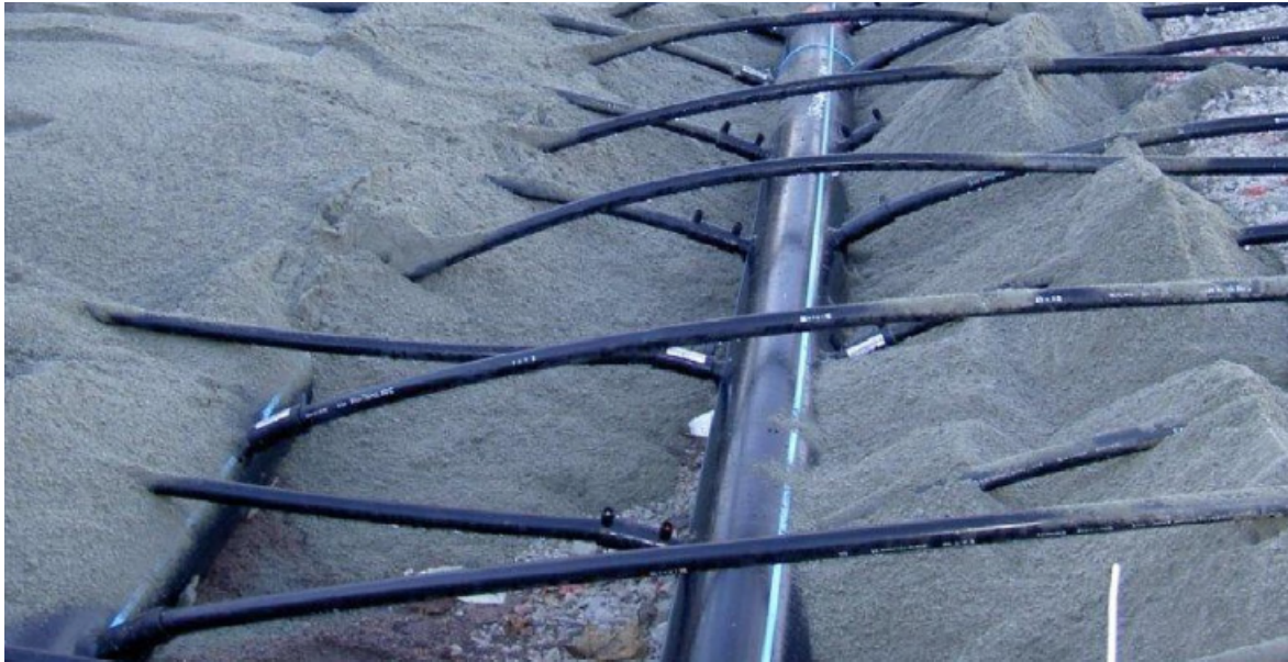
Figure 14: Example of manifolds for flow distribution to many loops in parallel (LK Systems)
