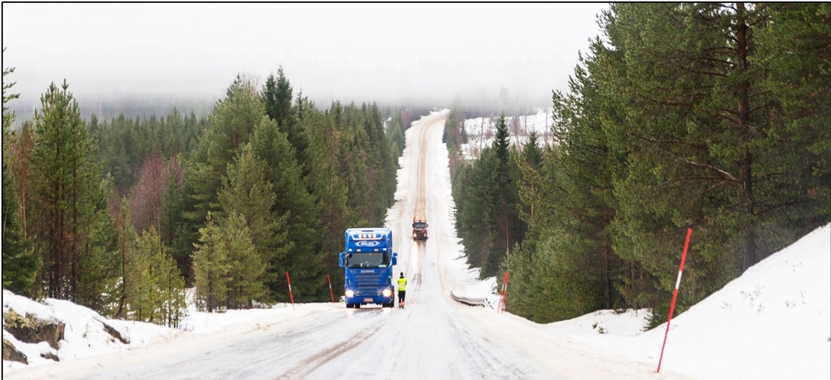
Figur:10: "Göteborgsbacken" prior to installation of the HHP system (Tidningen Energi 2020-03-19)
